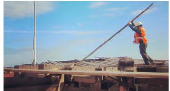
A contractor lifting a piece of decking that will be salvaged.
