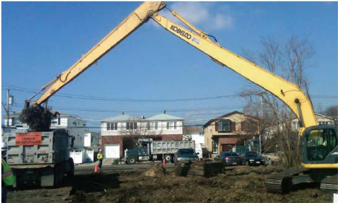
Crews working to remove debris from the Oakwood Beach wetland in Staten Island.
