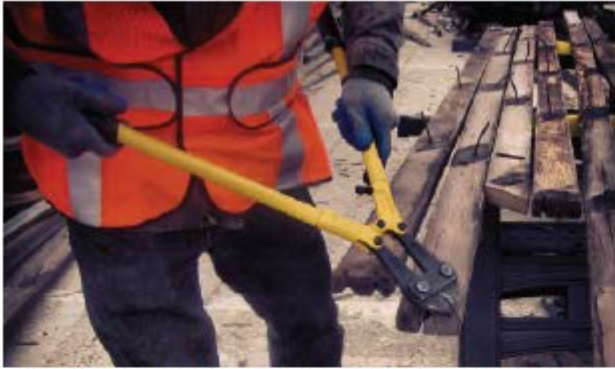
Contractors removing nails from wood to be salvaged from the Rockaway Beach boardwalk.
