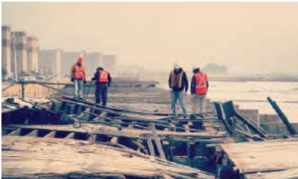
Contractors working on the Rockaway Beach boardwalk.
