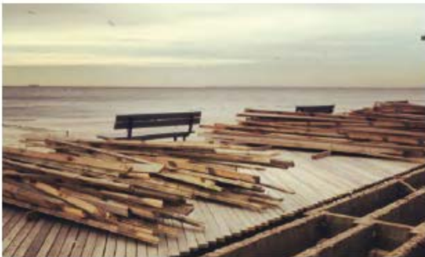
Stacks of boardwalk decking that will be recycled.
